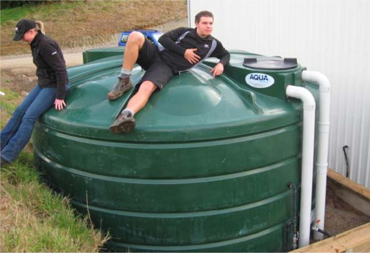
This storm water tank roughly collects 17,500 litres per month of water from the roof of our new work shop. The water will be used to wash vehicles as this is our highest water consumption within the site.
